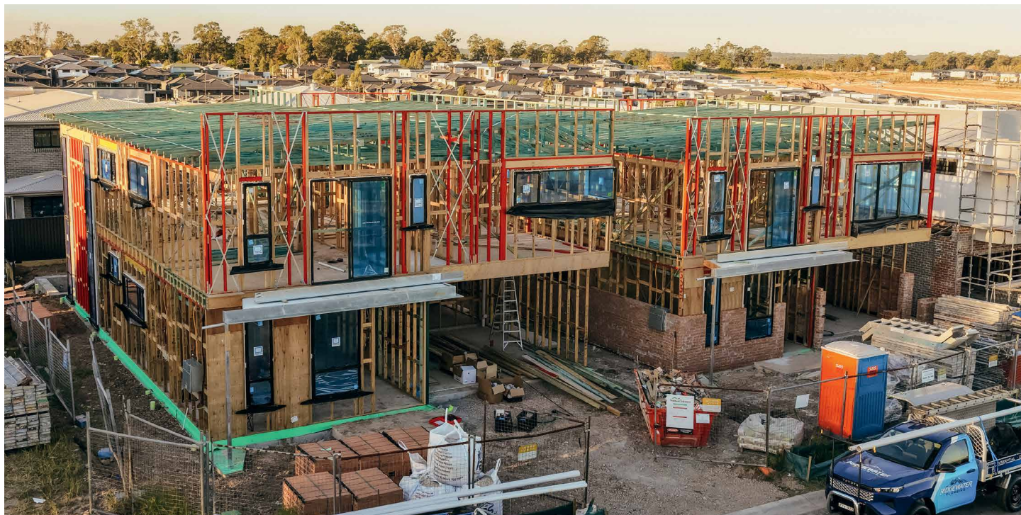
Above: The suite of Spec EWP products were specifically requested for 2 side-by-side builds in Sydney's North West.
