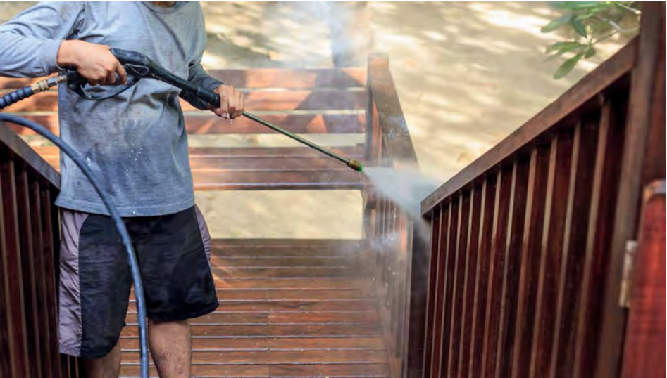
Above: Specialist product and a high-pressure hose can repair surface stains on an old deck.
