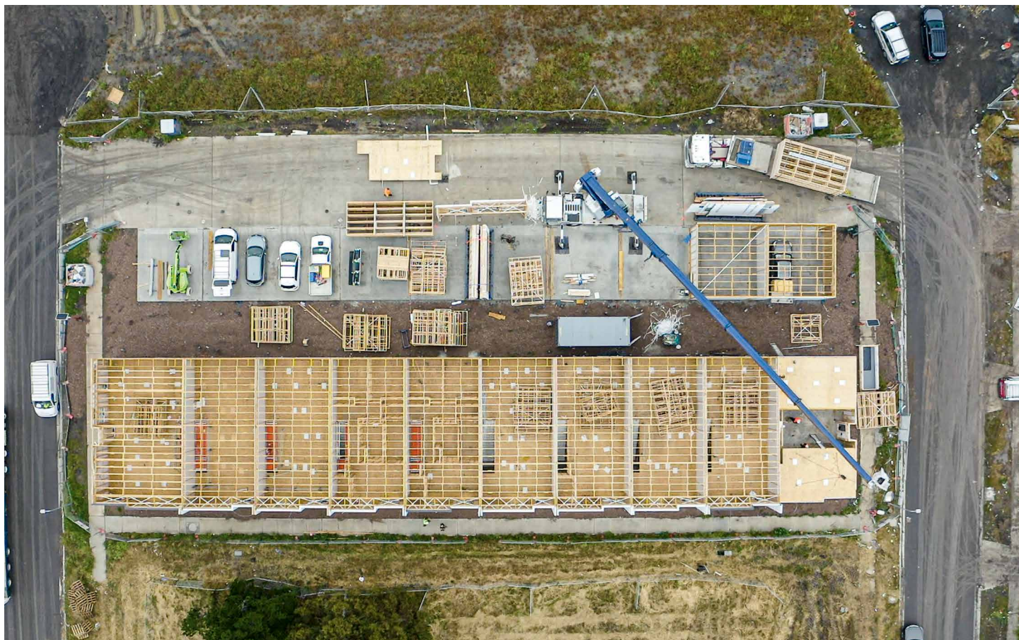
Above: The repeatability of timber elements in multires, both townhouses such as this TBS build at Kalkallo and apartments, delivers manufacturing economies and buildings that are faster and easier to assemble.
