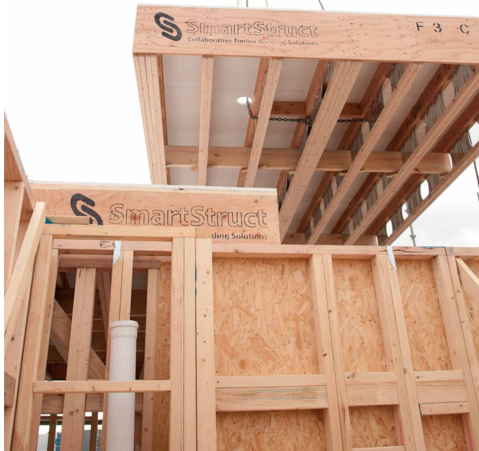
Above: Panel- and cassette-based construction also removes a lot of working at height, making sites safer.
