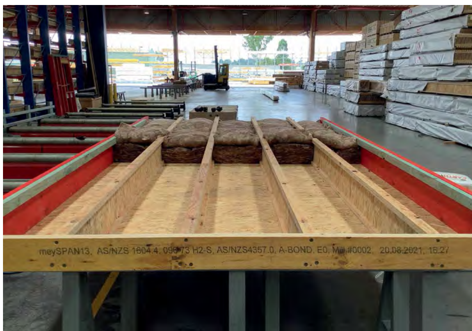
Above: Closed cassettes for Blue Eco Homes also include insulation, finished with a watertight membrane.
