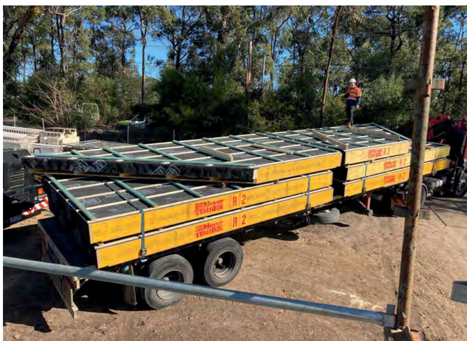
Above: Both closed and open roof cassettes fit onto a standard truck for delivery.
