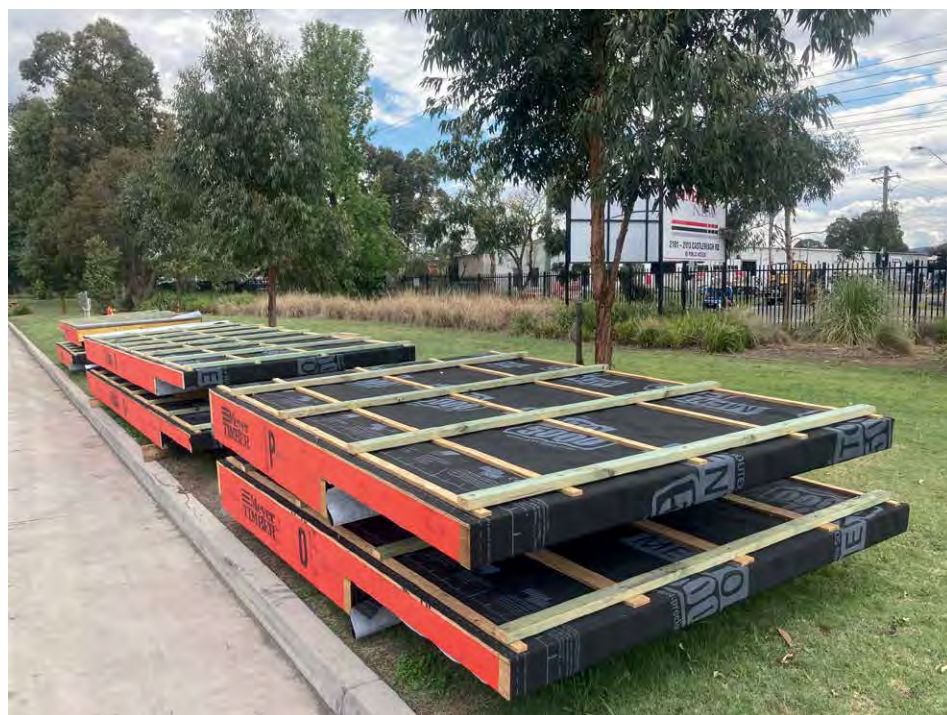
Above: Meyer's closed roof panels manufactured for Blue Eco Homes.
