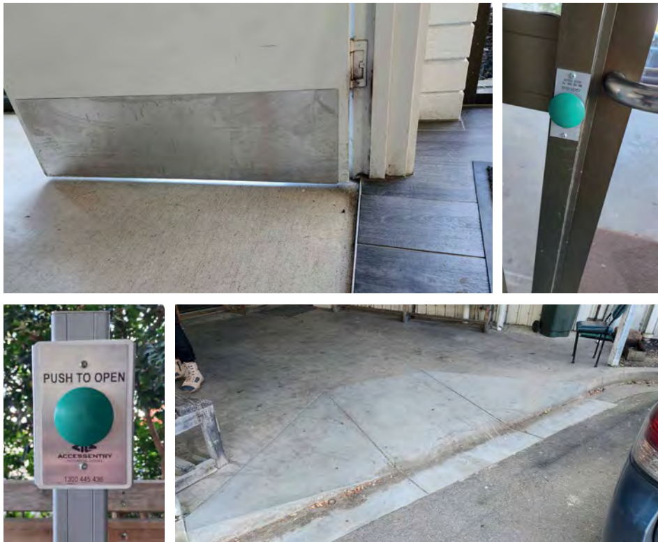
Above: Simple modifications like electronic doors and ramps at Alpine Truss were supported by JobAccess.
