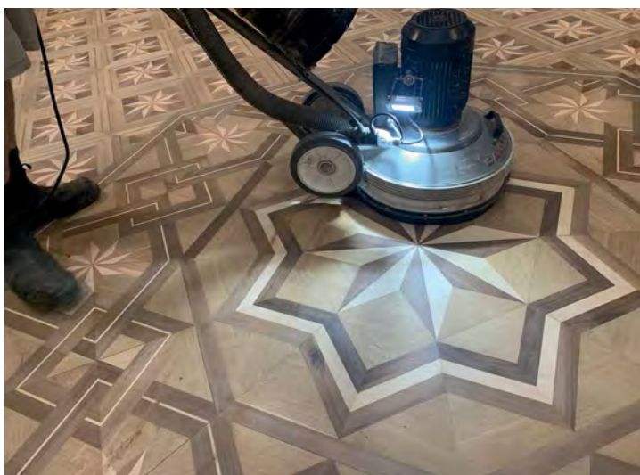
Above: The refinishing process uses multiple machines and grades of abrasive to first remove scratches and other imperfections in the parquet before polishing it to a smooth level finish. Finally, a protective coating is applied manually to both let the floor shine and feed the timber parquets.
