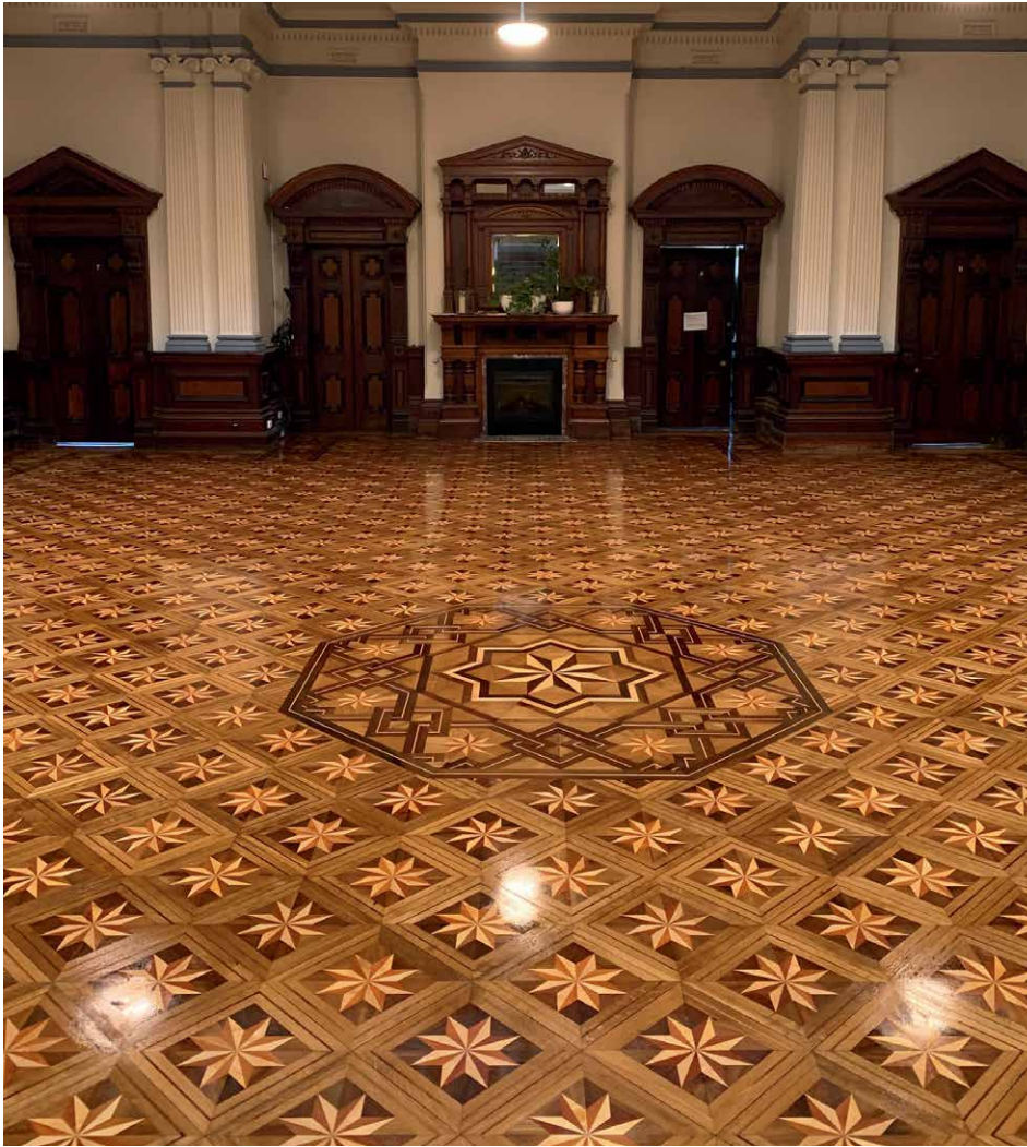
Above: The completed floor after its careful process of restoration, sanding, polishing and oiling. It was originally laid by Italian craftsmen using European walnut, oak and sycamore.
