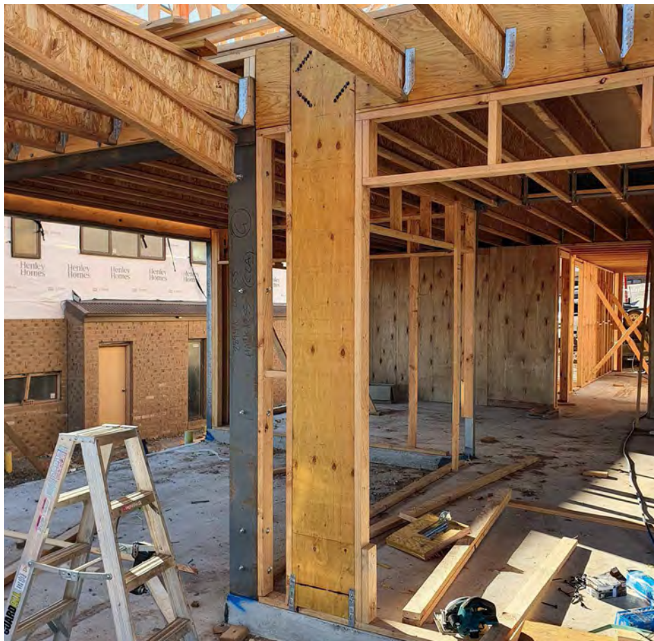
Above: The finished installation of meyBRACE from the solution planned in the image below.
