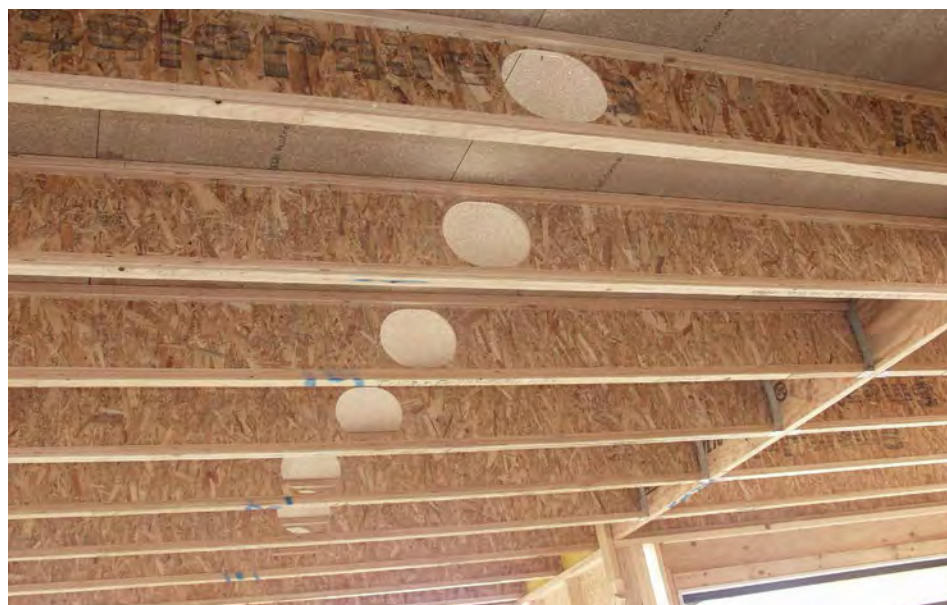
Above: SmartJoist with holes pre-cut for services. It's a hugely popular product and will now be made locally.
