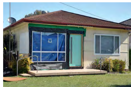
Above: Fibro sheeting and boards found under eaves and as linings are places you might expect to find asbestos, but it can also be in the adhesives and seals.
