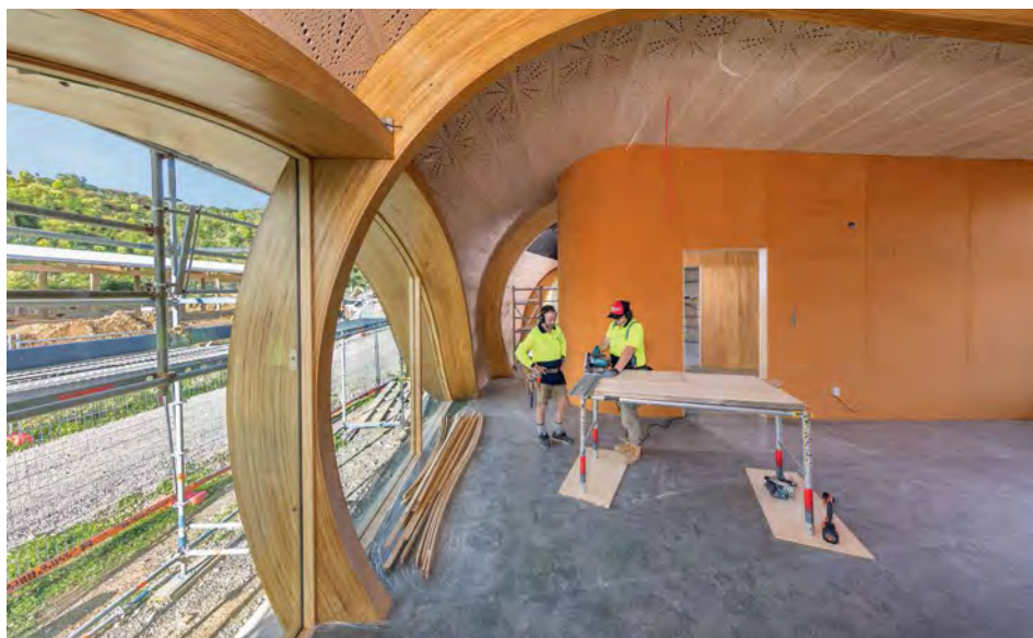
Above: Green School: delivery and assembly of the curved glulam members was surprisingly quick.
