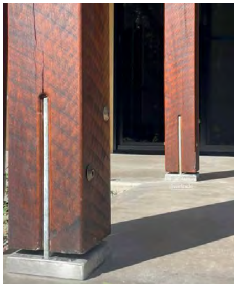
Above: VUETRADE's T-blade system shows minimal steel, delivering a tidy, safe connector that highlights the real visual hero of the design: the timber.
