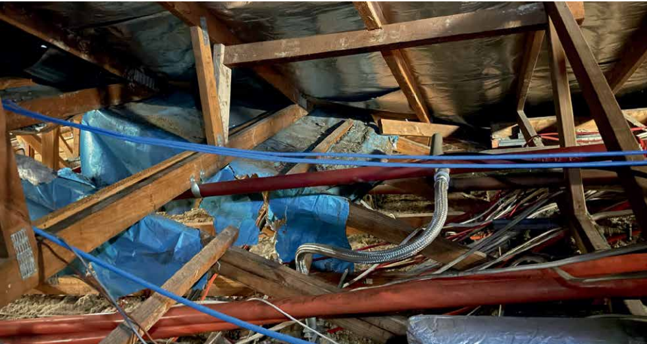
Above: This tangle of services in the roof of an aged care home adds load that needs specific designs.
