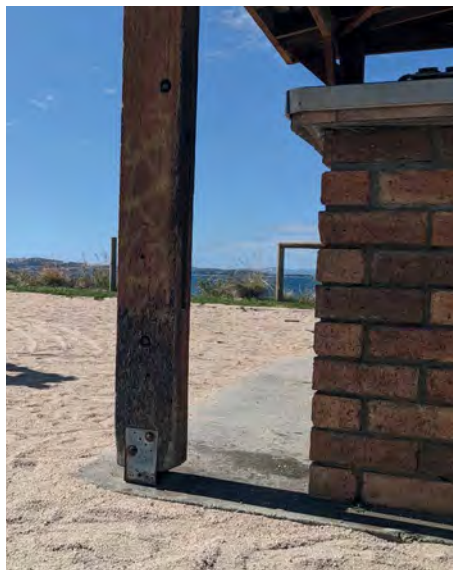
Above: Galvanised products aren't suitable for coastal sites like this picnic shelter as they rust and let rot into surrounding timbers. VUETRADE has often been called in to replace product like this with stainless steel.
