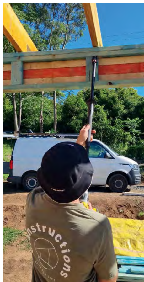
Above: Installing Simpson truss screws using a Quik Stik, eliminating the need to work at height.
